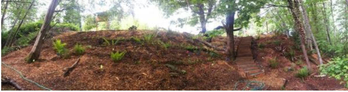
Figure 2: Polygon 1 after the waste pile removal and restoration
