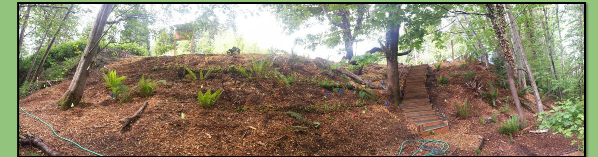
Panoramic view of slope stabilized with living fascines as well as sword fern plantings.
