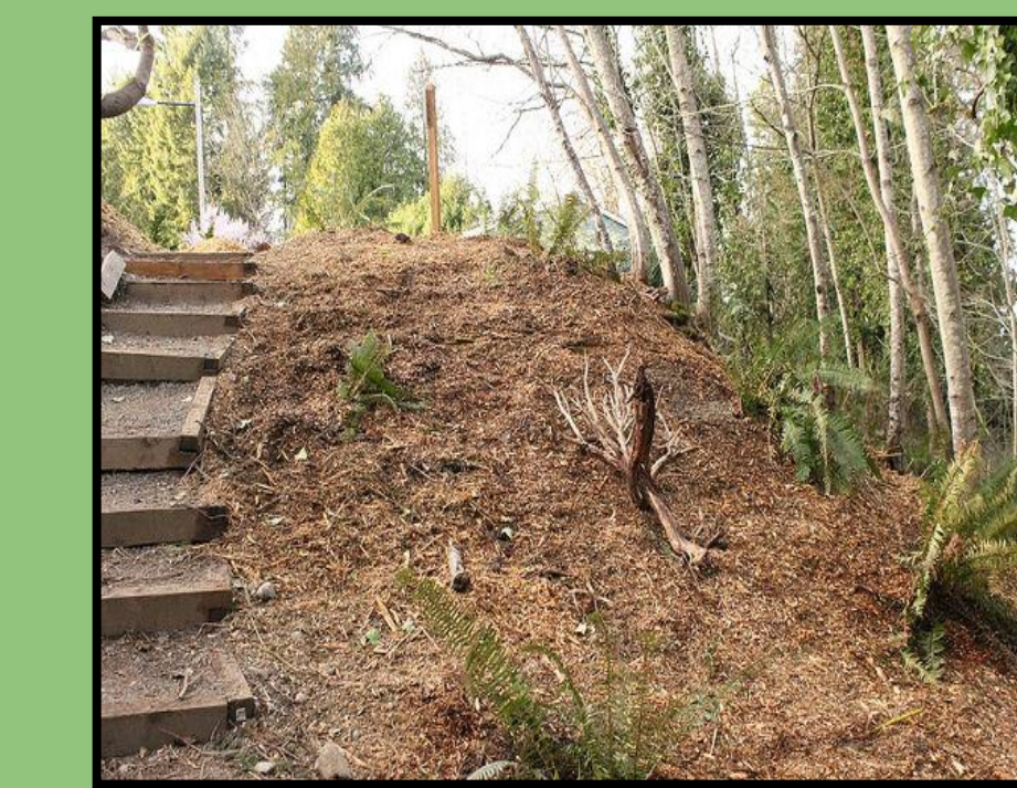
Left: Installed stairs and fascines, removed ivy and stabilized hillside. Right: Installed wattles and red-osier dogwood live stakes.
