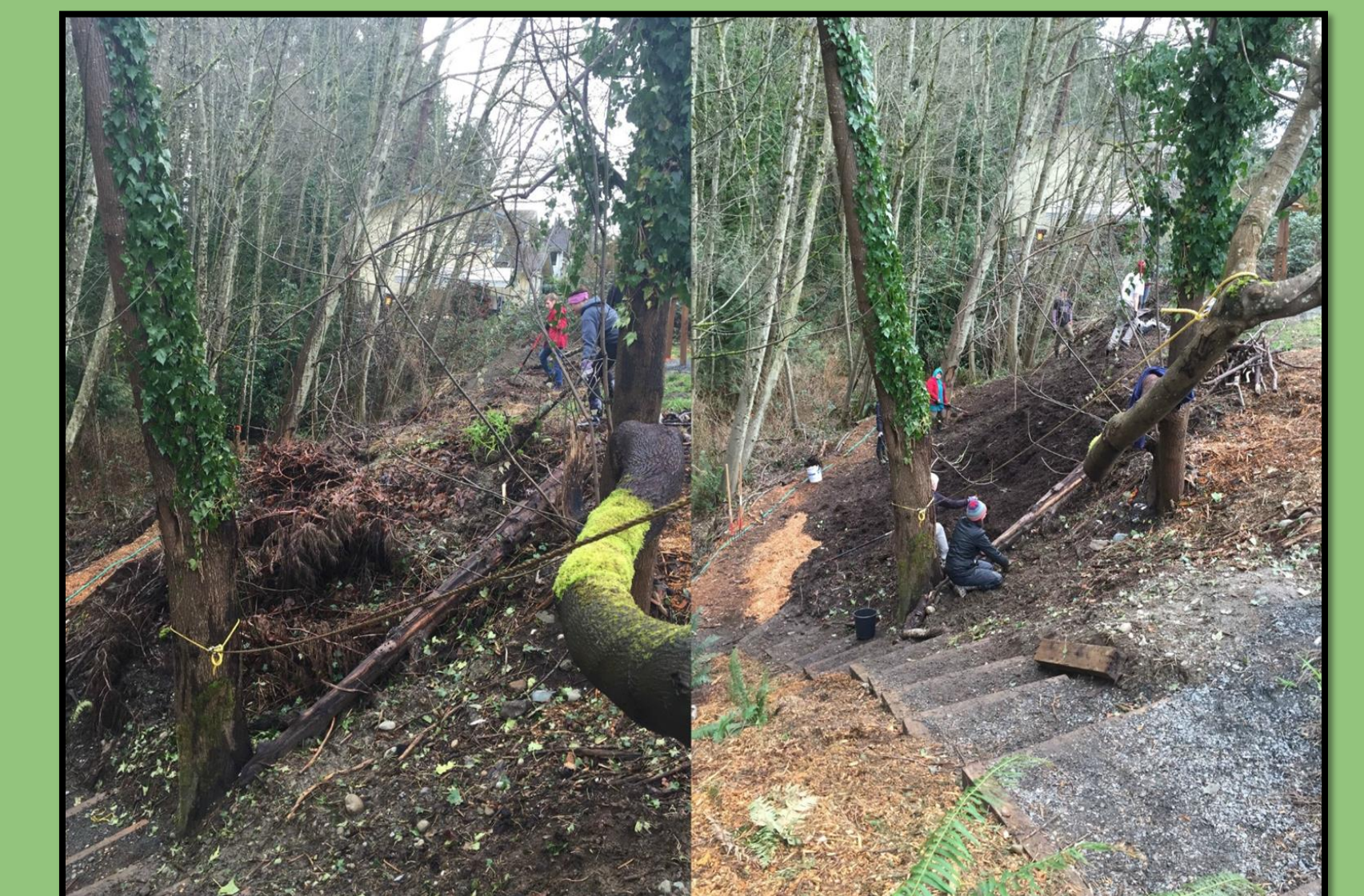
Left: Installed stairs and fascines, removed ivy and stabilized hillside. Right: Installed wattles and red-osier dogwood live stakes.
